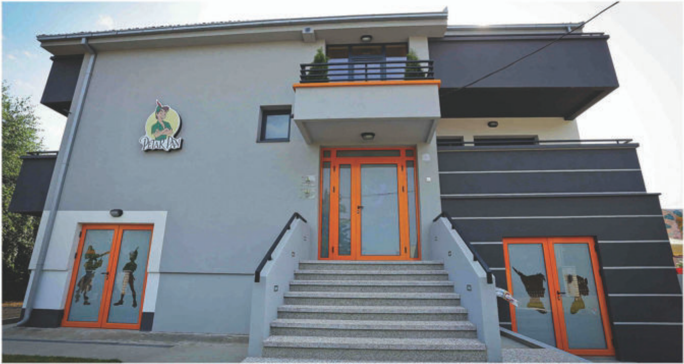
Kindergarten, Kragujevac, Serbia Kindergarden, Kragujevac, Serbia
